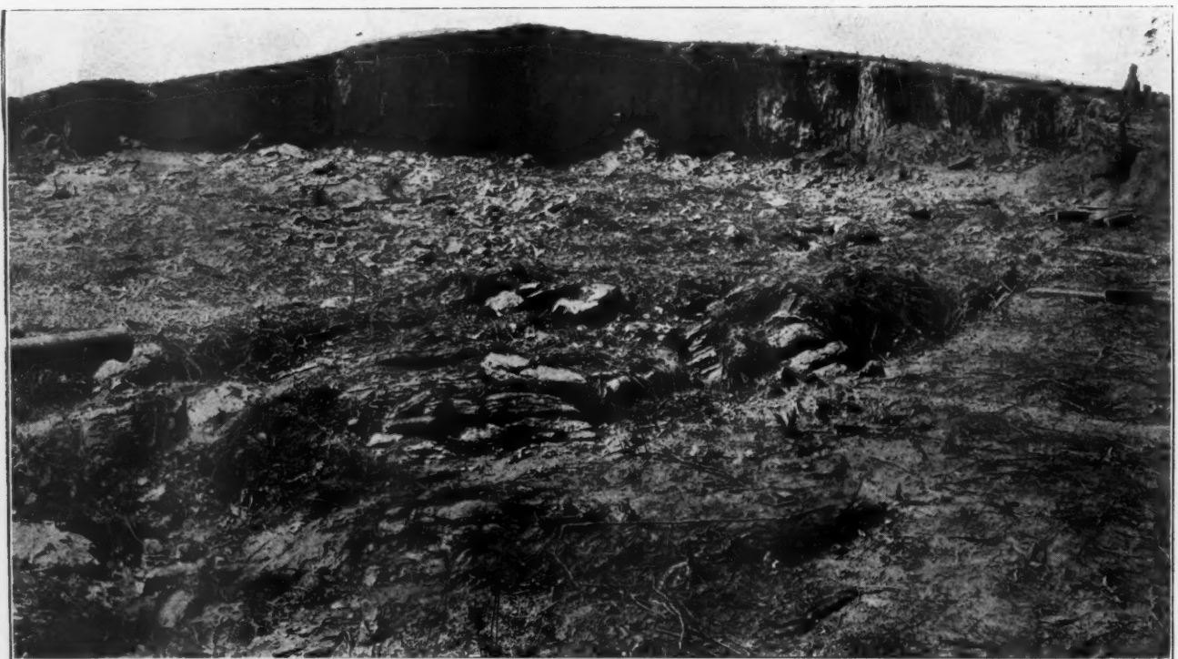
Showing the Progress of Hydraulic Stripping
